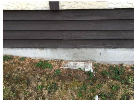
View of foundation
