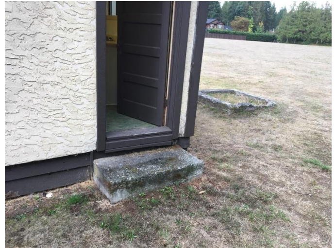
View of rear kitchen door
