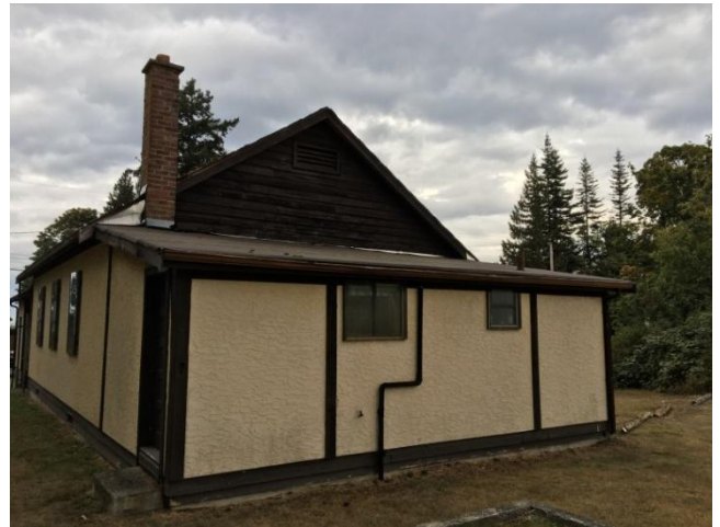
View of roof over rear of Hall
