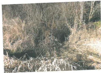
8(e): Ditch at discharge of north property ditch
