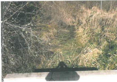
8(d): Ditch looking north at entrance
