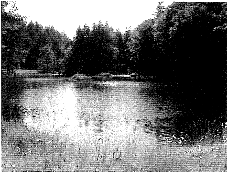
Photograph 2. View of pond from earthen dam.
