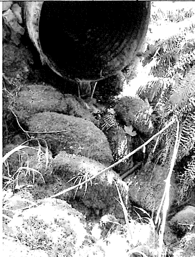
Photograph 4. June 2014. View of the outlet of the culvert at Taylor Bay Road.
