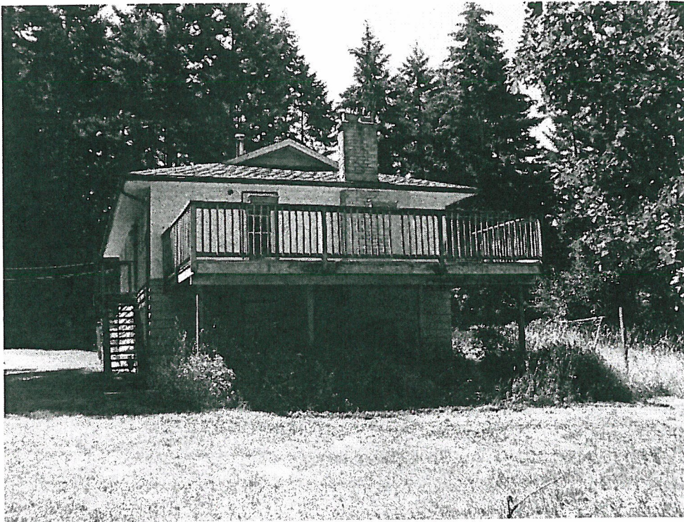
Photo #2 – Facing south, house with deck / carport and yard in foreground.
