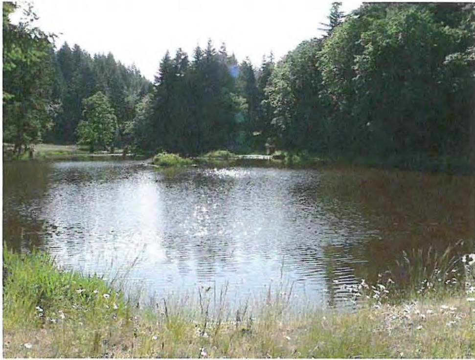
Photograph 7. View east from the dam to the upper end of the pond.
