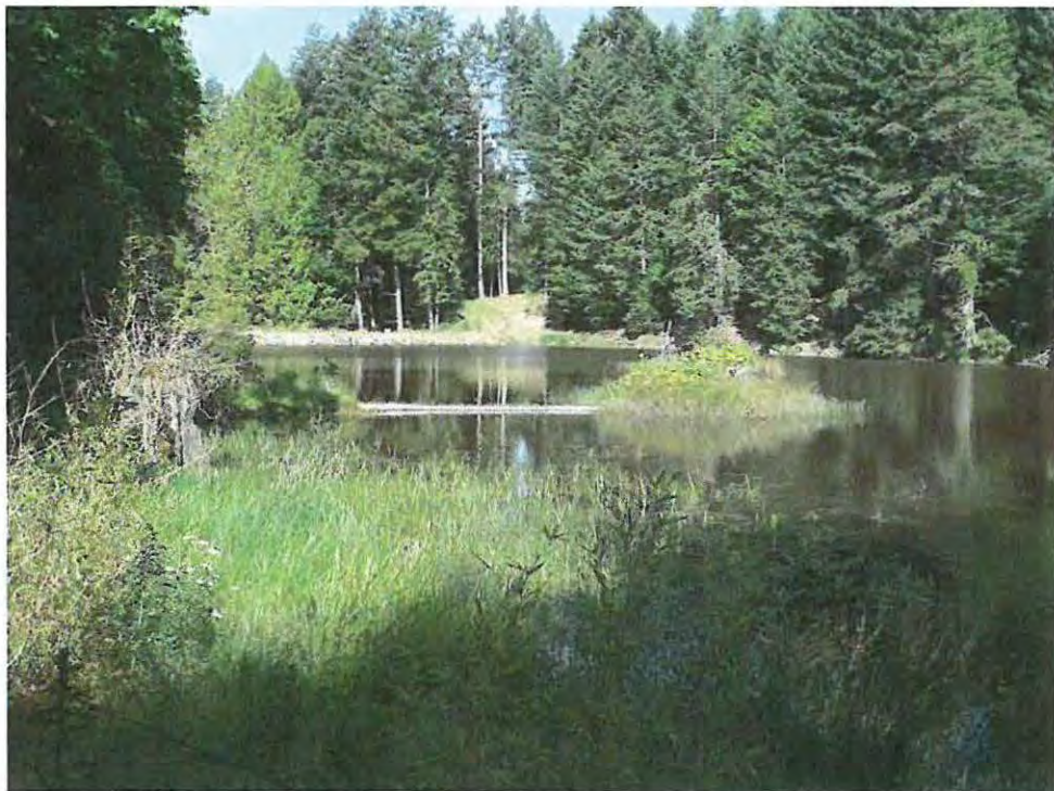
Photograph 8. View west from the south side of the pond to the dam.
