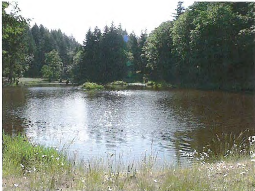
Photograph 2. View of pond from earthen dam.
