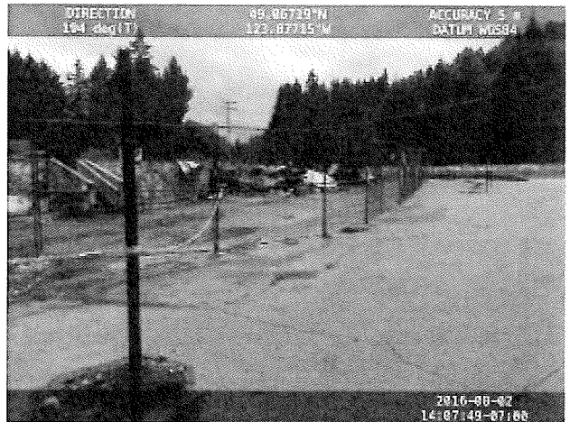
Open Foundation Structure
