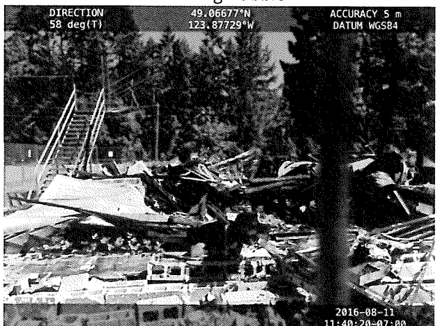
Freestanding Stair and Landing Remnant
