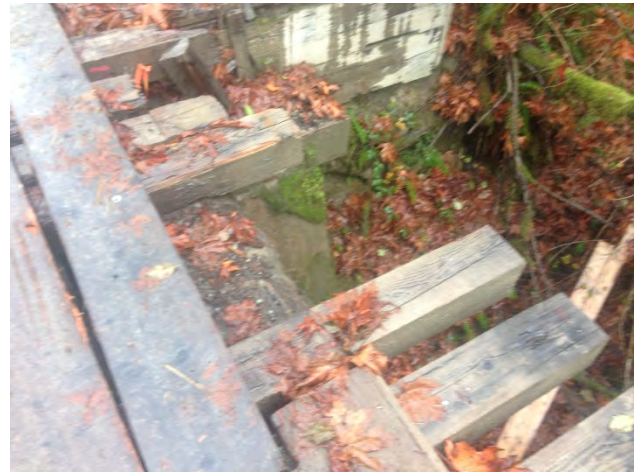
Deck near North Abutment
