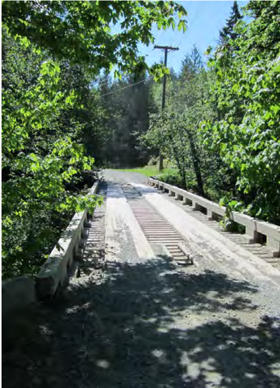
Figure 1. Haul bridge that crosses the river within the LQRRP.
