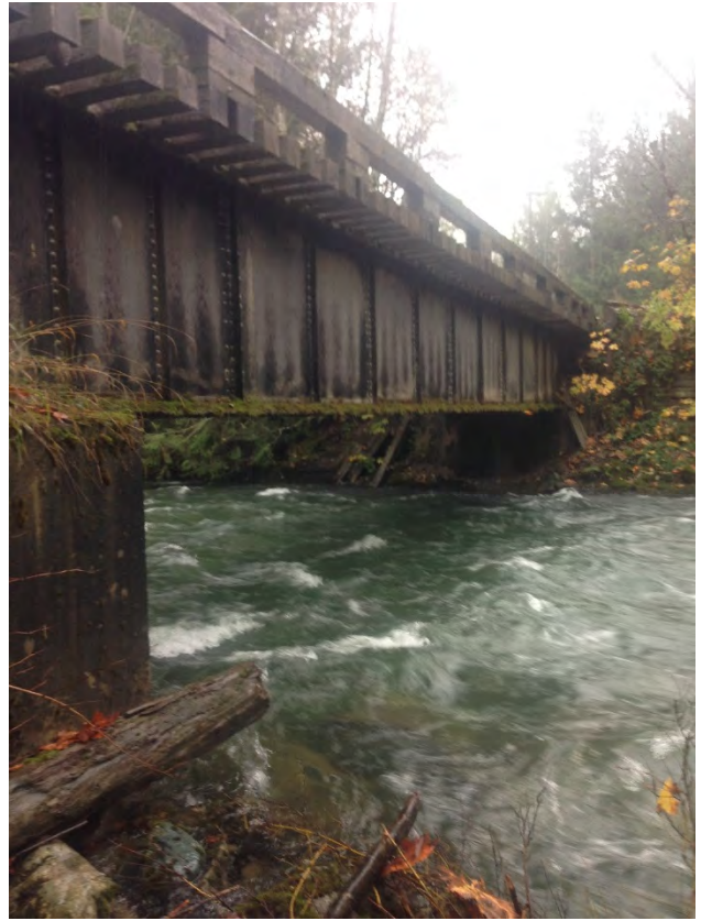
Main River Channel – Steel Girder Span
