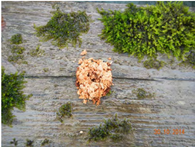
Drill sampling - shavings from top of barrier
