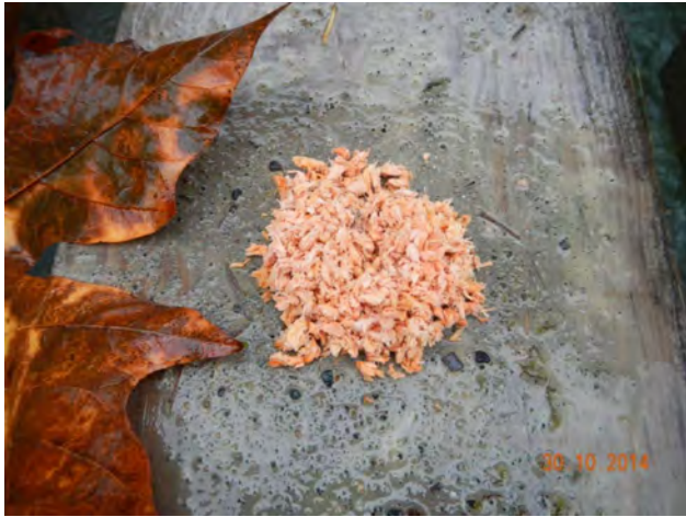
Drill sampling - shavings from top of barrier
