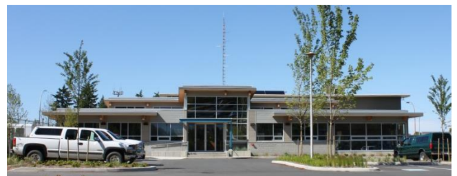
RDN Transit Admin Building
