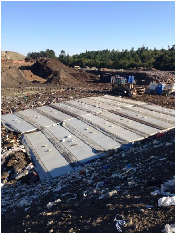
New cover system on active landfill
