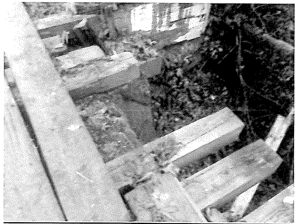
Deck near North Abutment
