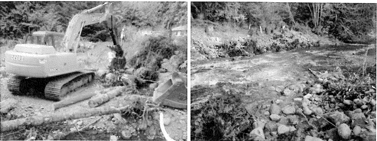
Restoring the eroded bank and post-treatment.
