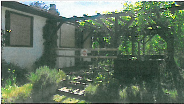
west side entrance and arbour
