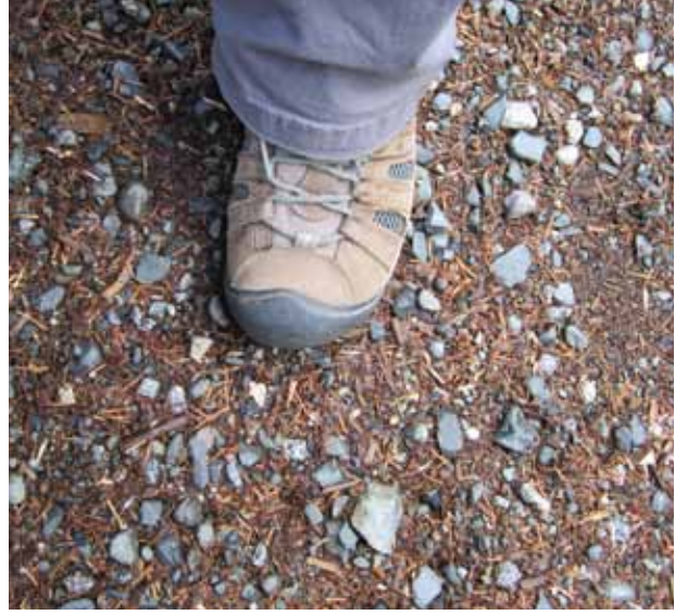
Trail surface of gravel and bark mixture
