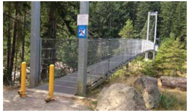
Steel bridge at the Top Bridge Regional Trail
