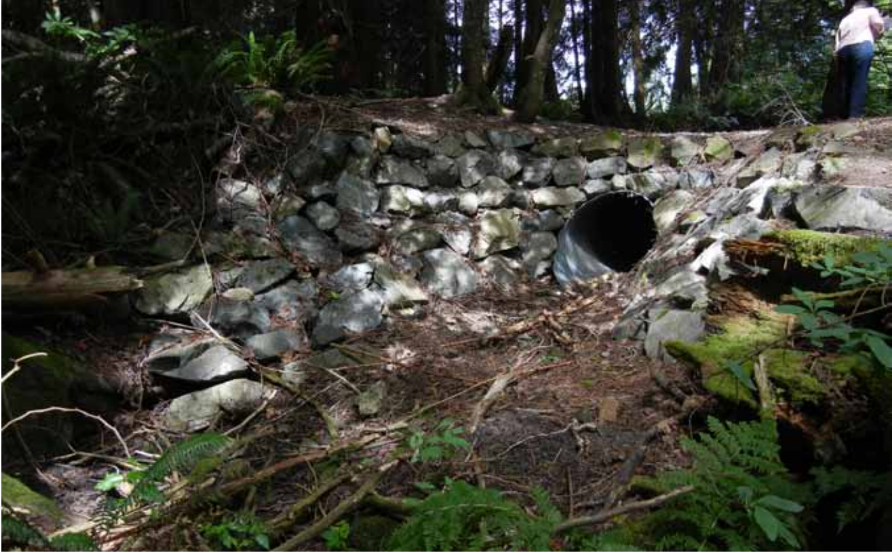
Culvert under trail
