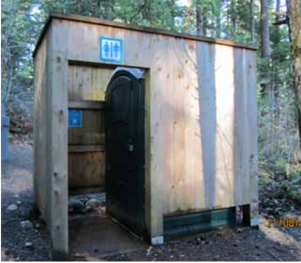
Portable toilet with surround
