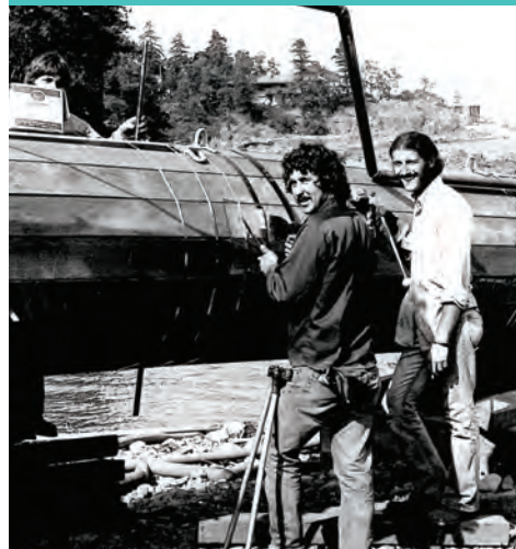
INSTALLATION OF THE ORIGINAL GREATER NANAIMO POLLUTION CONTROL CENTRE OUTFALL IN 1974.
