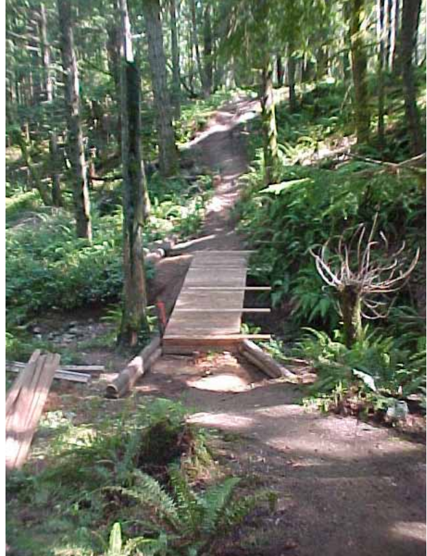
Footbridge under repair
