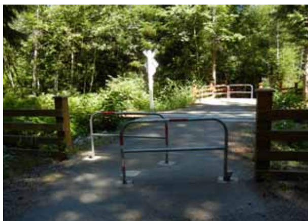
Accessible railroad baffles
