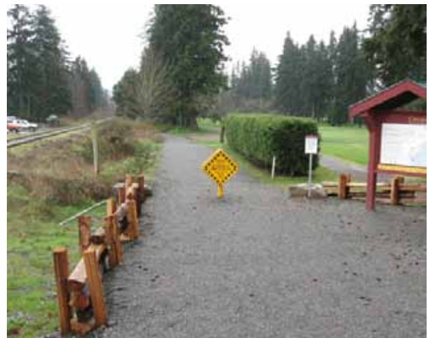
E&N Rail trail in CVRD
