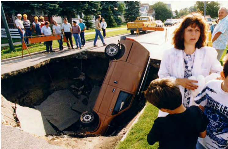
Figure 2. A sink hole caused by a watermain break adjacent to a poorly maintained sewer
