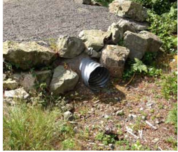
Culvert under parking area
