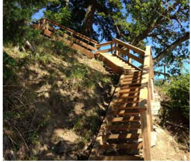
Engineered stairs to beach area
