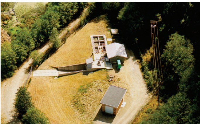
NANOOSE BAY POLLUTION CONTROL CENTRE
