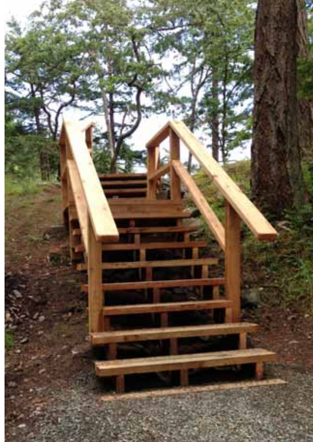
Stairs constructed with stringers from demolition project
