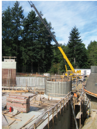
CONSTRUCTION OF THE DIGESTERS AT THE GREATER NANAIMO POLLUTION CONTROL CENTRE
