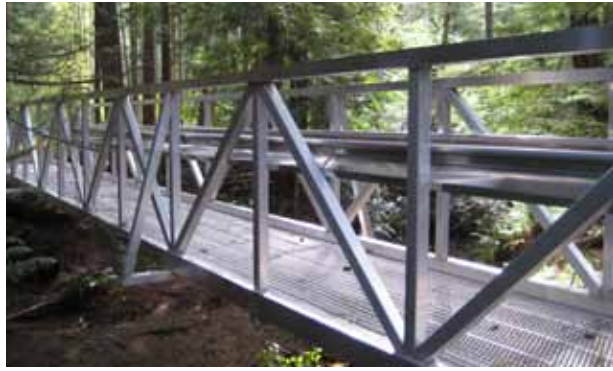
Steel bridge at the Lighthouse Regional Country Trail
