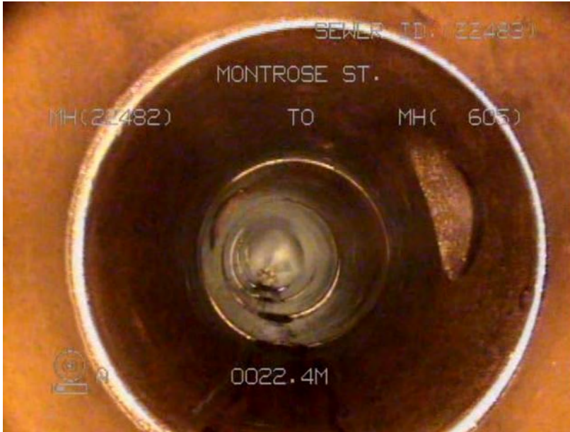
Figure 11. A sewer is collapsing and is highly likely have infiltration issues
