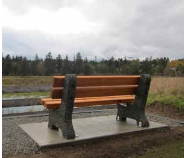
Concrete bench with cedar slats
