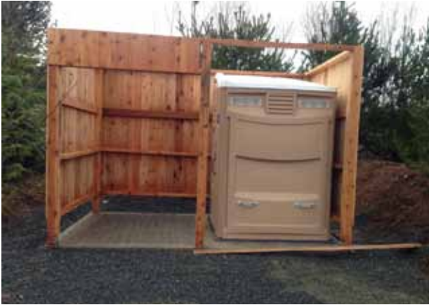
Accessible toilet surround construction
