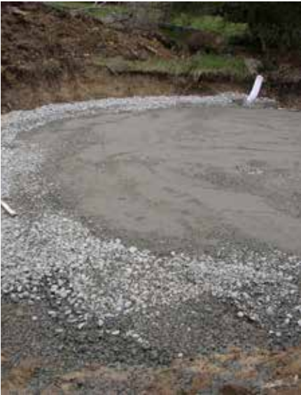
Compacted tank pad for steel cistern.
