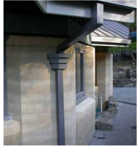
Custom-designed debris catchment box.
