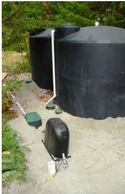
Tank manifold pipe and valve boxes after backfilling.
