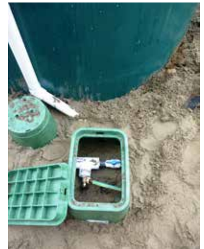
Partially backfilled valve boxes.
