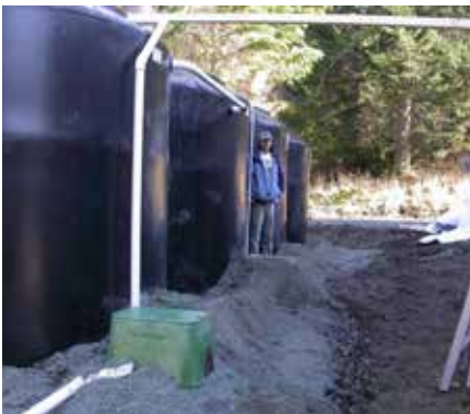
Four poly 11,365 L (2500 gal) tanks, partly backfilled.
