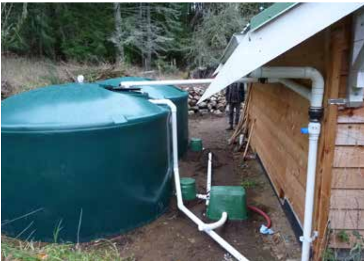
Two 1660 gal (7,550L) poly tanks with interconnecting piping and protective valve boxes (before final backfill).
