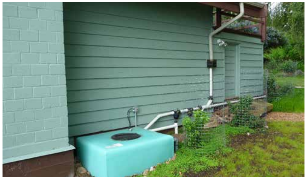
Dry triple-cleaning system to surge/pump tank, downspout to debris box, and a pair of Banjo screen mesh gravity filters.
