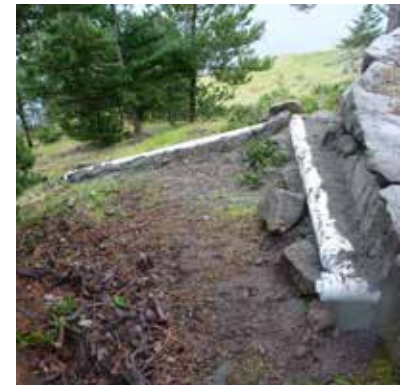
Large, underground FFD pipe partly backfilled.
