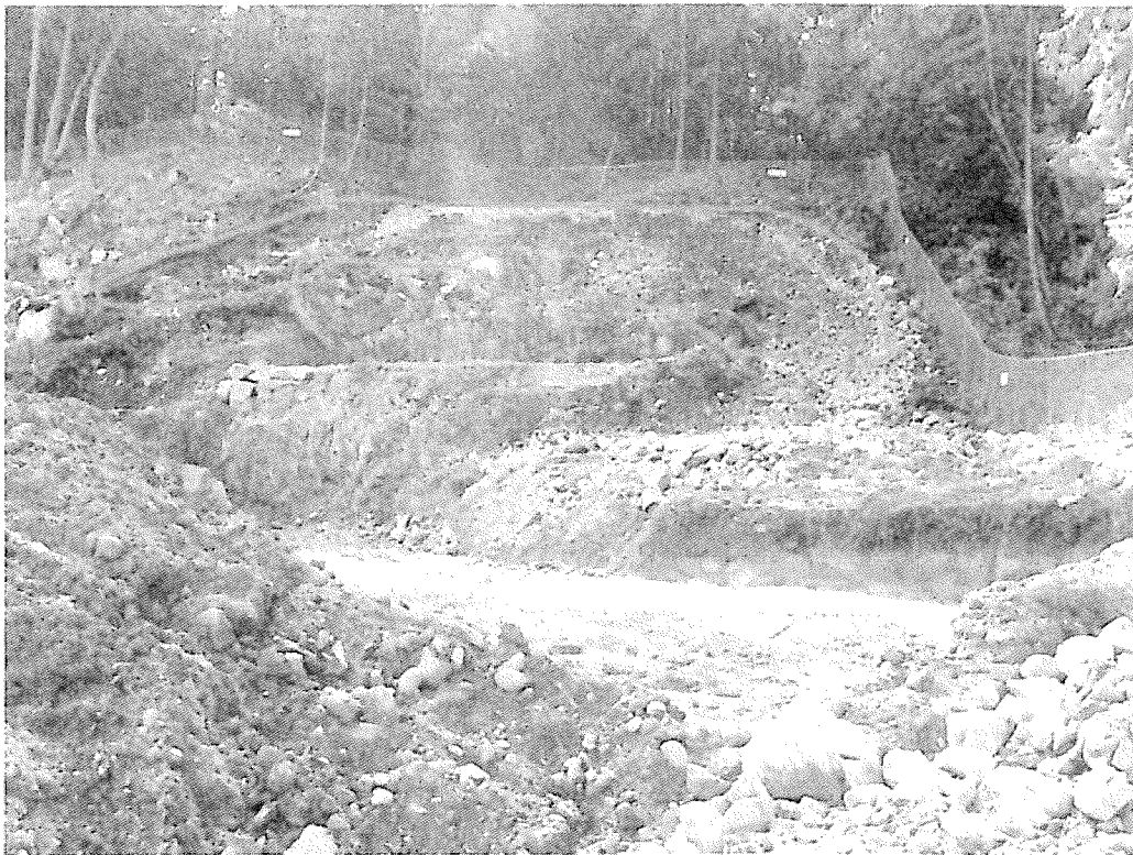
Photograph 1. View south from Andover Road to recommended revegetation area.
