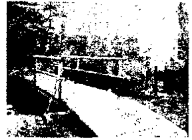
21 Counting Station Bridge
