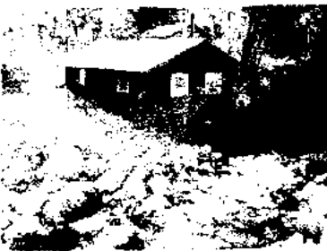
⑦ Hatchery Building 1
