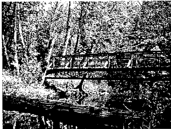
Morden Colliery Regional Trail – Thatcher Creek bridge
