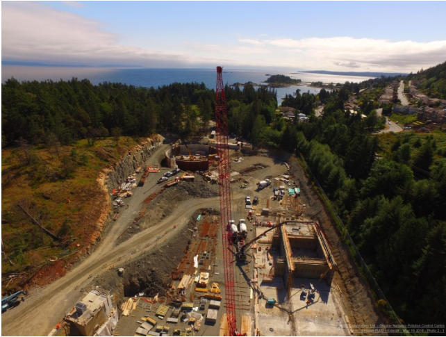
Photo left: Secondary treatment construction area
