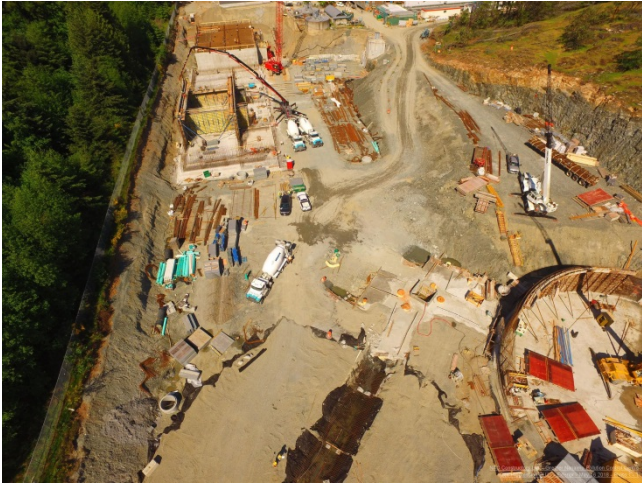
Photo right: Secondary treatment construction area
