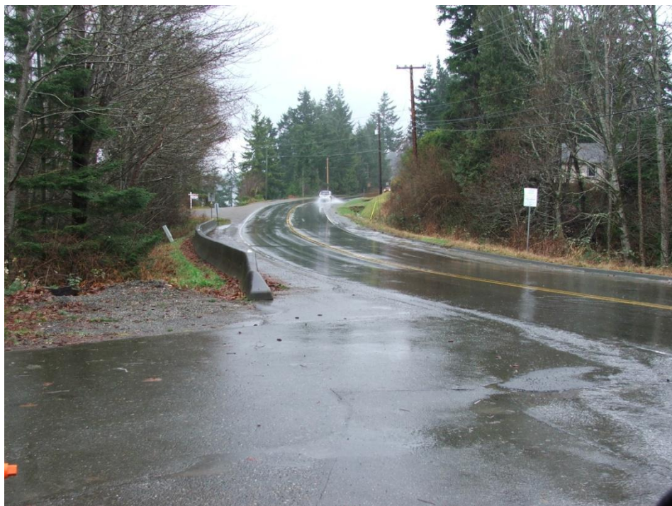
Thames Creek Crossing (Looking Southwards)
