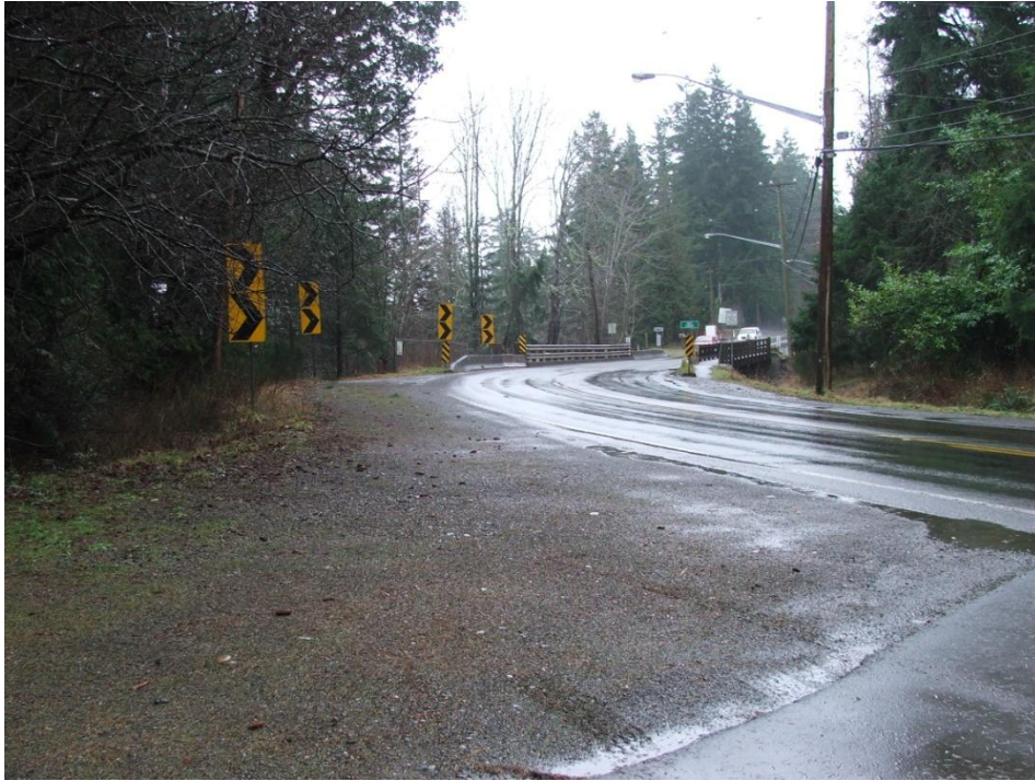
Nile Creek Bridge (Looking Southwards)
