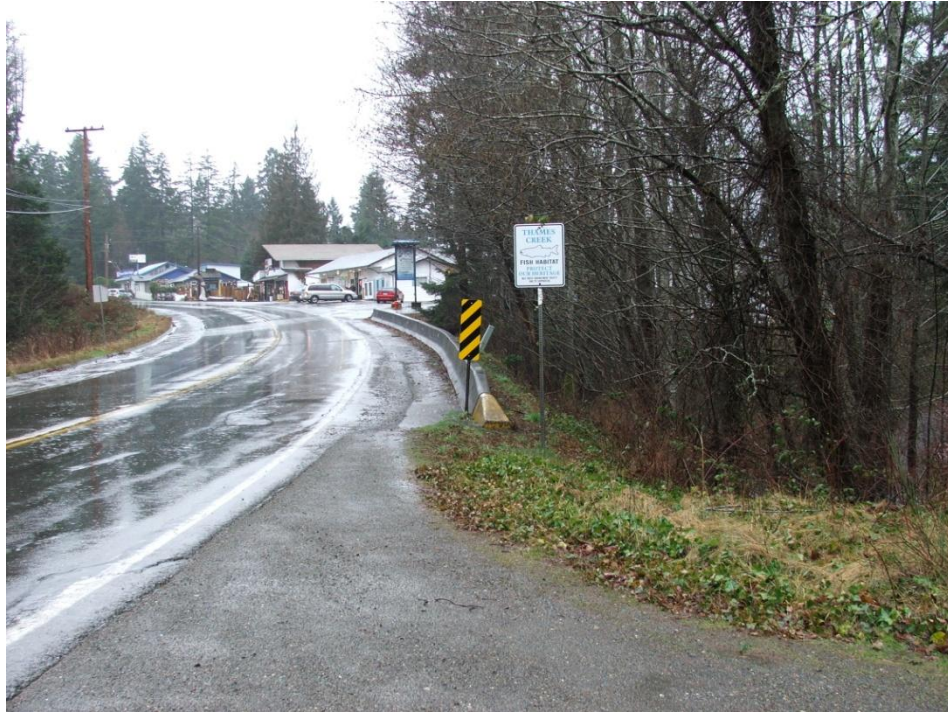
Thames Creek Crossing (Looking Northwards)
