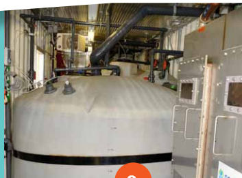
Waste water from the CRTS is treated at the on-site treatment plant and reused for floor washing in the transfer building.
