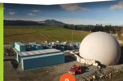
Methane from the landfill is used to generate electricity.
