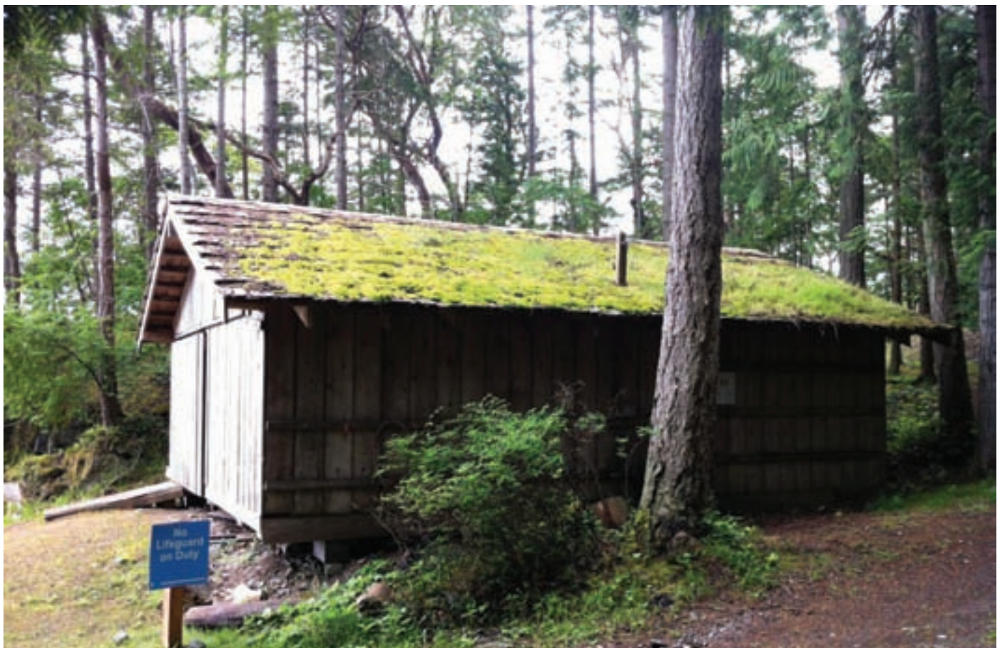
Figure 15. The Boat House - Typical building condition
