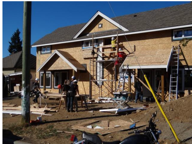
VIU Carpentry Program students volunteering at a Nanaimo Habitat Duplex Site
