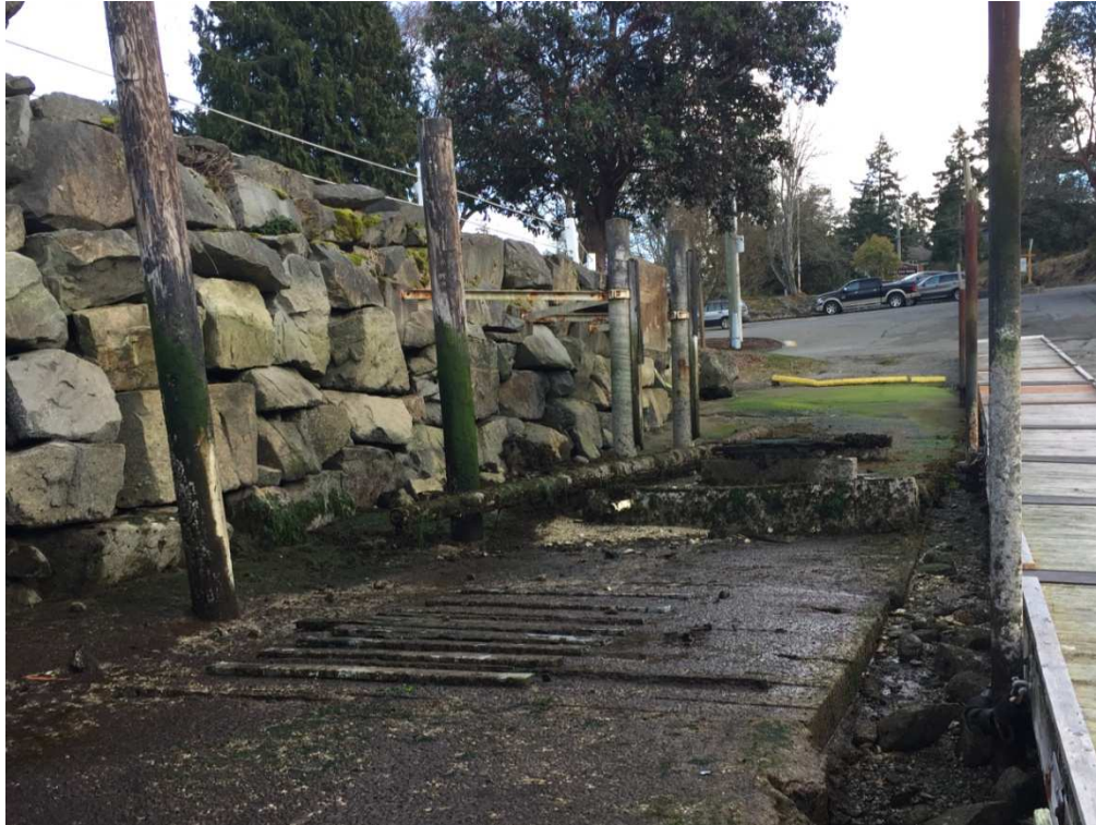
Figure 9. Boat cleaning grid in the boat ramp area of Schooner Cove.
