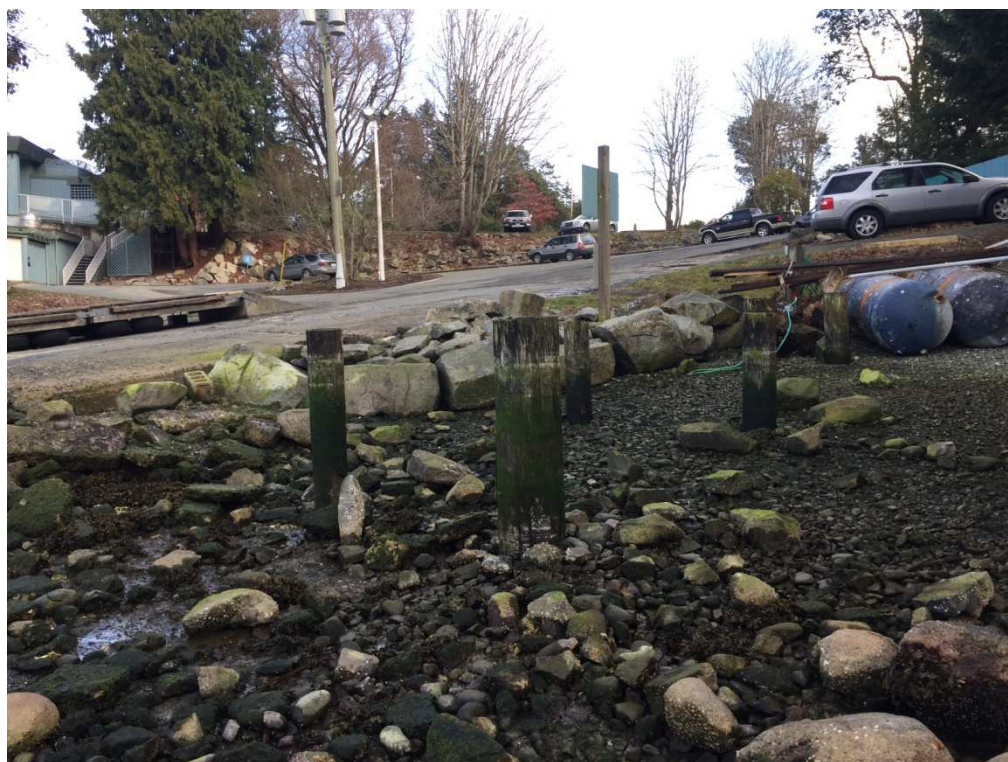
Figure 10. Piles to the west of boat ramp in Schooner Cove.
