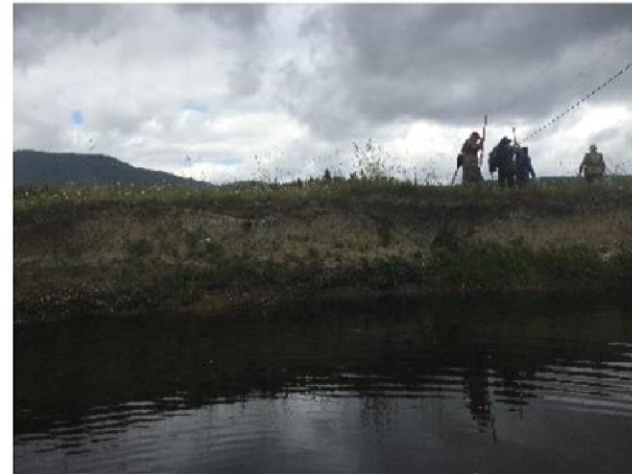
Reach 7 - erosion at bridge outlet
