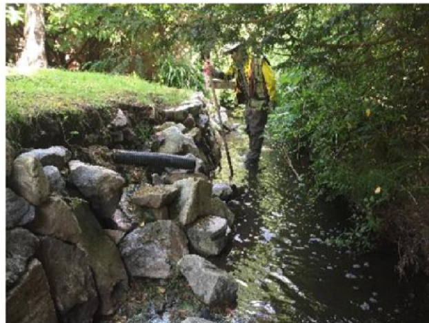
Metral M1 - altered bank and drains
