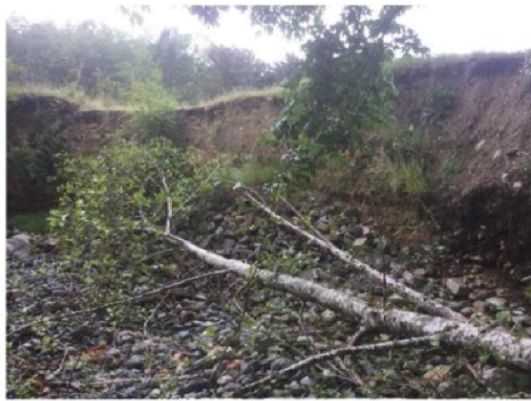
Reach 5 - Erosion site
