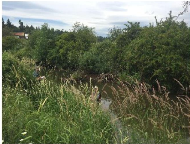
Reach 4 - eroding soil blocks
