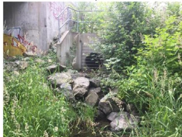
Reach 3 - Outfall into creek
