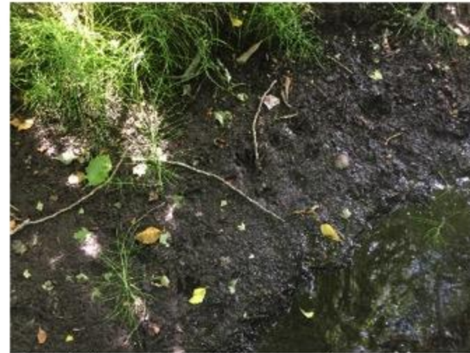
Photo 4) Accumulated sediments, erosion and raccoon tracks
