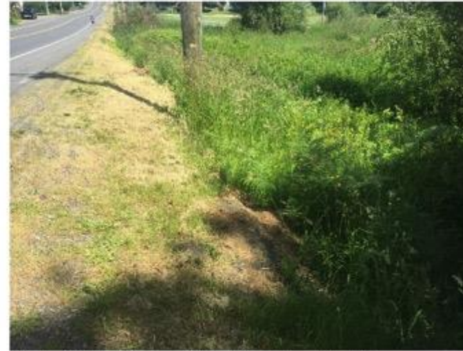
Photo 4) R1, Compost dumping along Park Avenue
