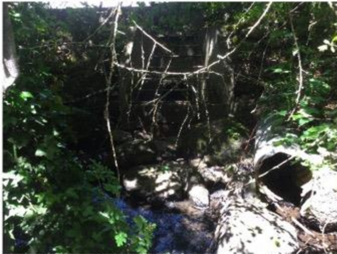
Photo 3) Two culverts draining from Beaconsfield Road
