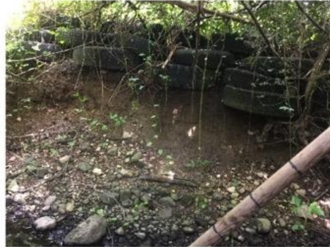
Photo 2) R3, Right bank reinforced with old tires
