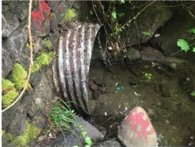
Photo 1) Culvert outlet below VIU
