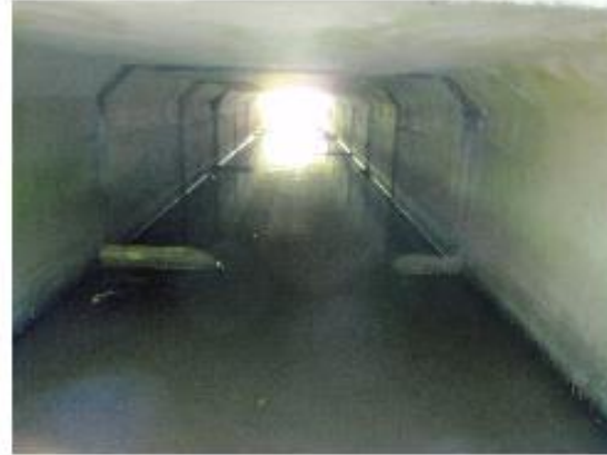
2). Culvert in Reach 4
