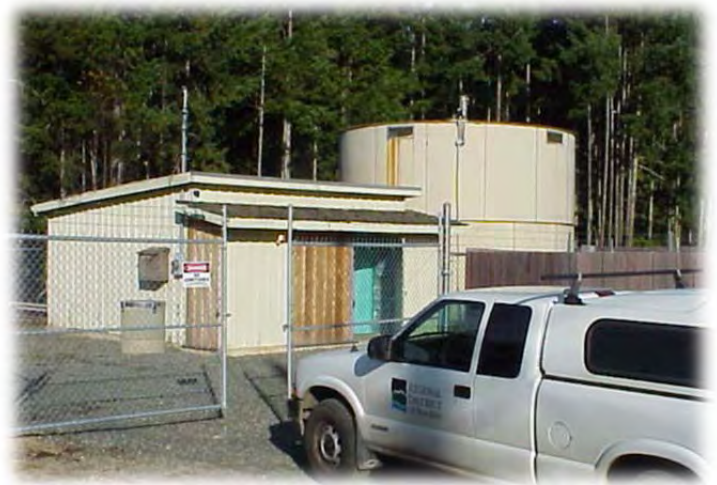
Melrose Pumphouse and Reservoir
