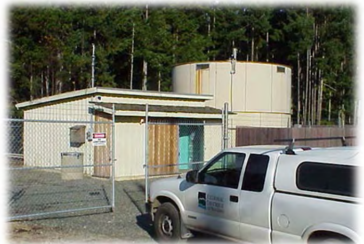
Melrose Pumphouse and Reservoir
