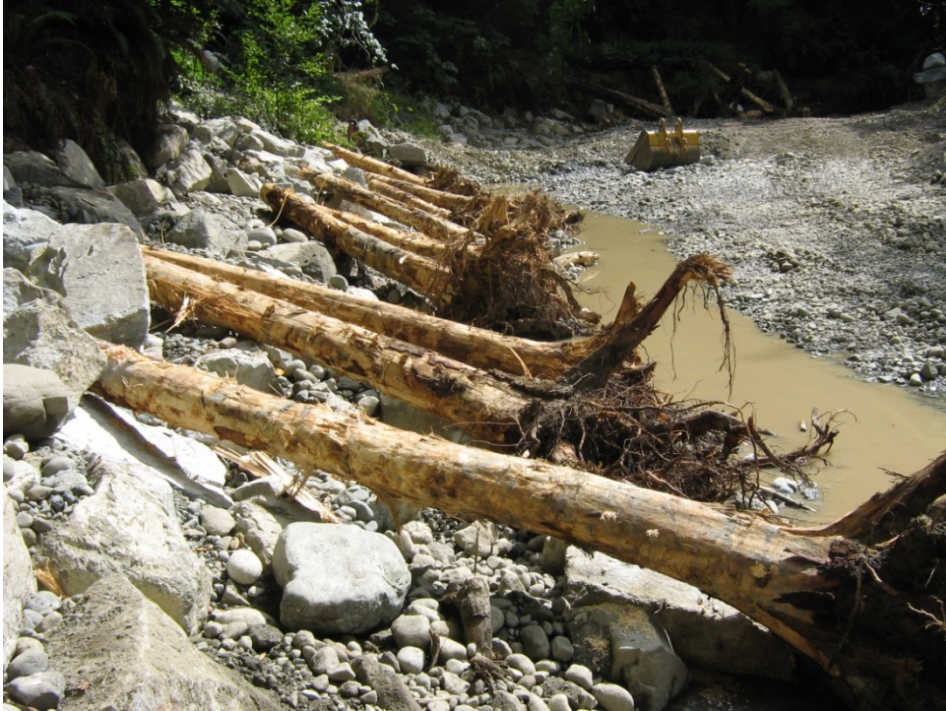
Photo 8. LWD was added to the linear riprap section to improve fish habitat values.
