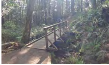
Footbridge on the north access route.
