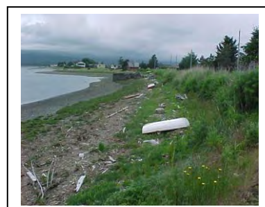
Beach and slope view west
