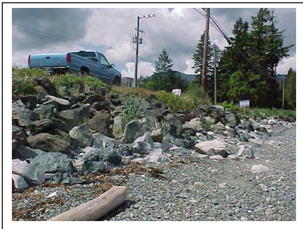
Riprap reinforced bank
