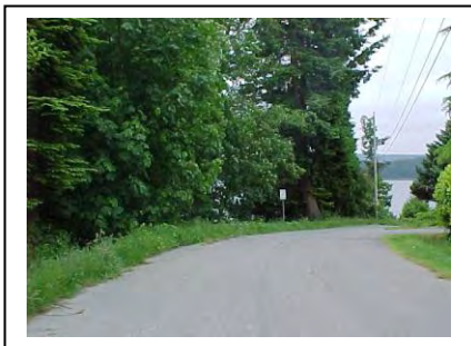
Seaview Drive and Shoreline Drive intersection. R/W on left
