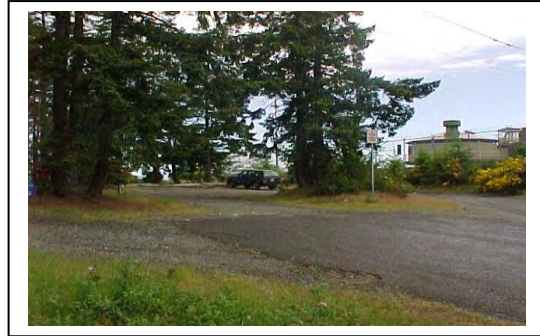
View showing Hydro structure
