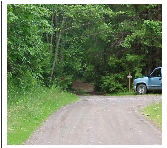
Intersection of Driftwood and Lasqueti Rds. Shows driveway entrance and R/W
