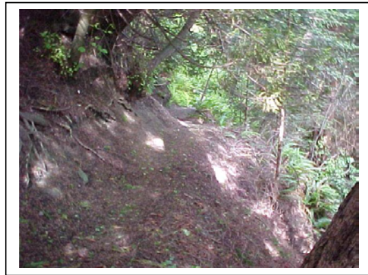
Mid main trail showing tread out slope and open side slope
