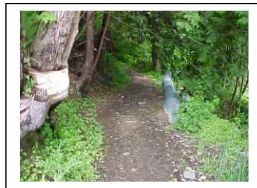
Upper trail with MoTH drainage culvert
