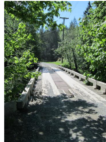
Figure 11. Haul bridge that crosses the river within the LQRRP.
