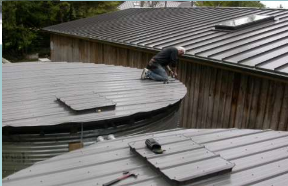
Wood-frame and steel roof with inspection hatch
