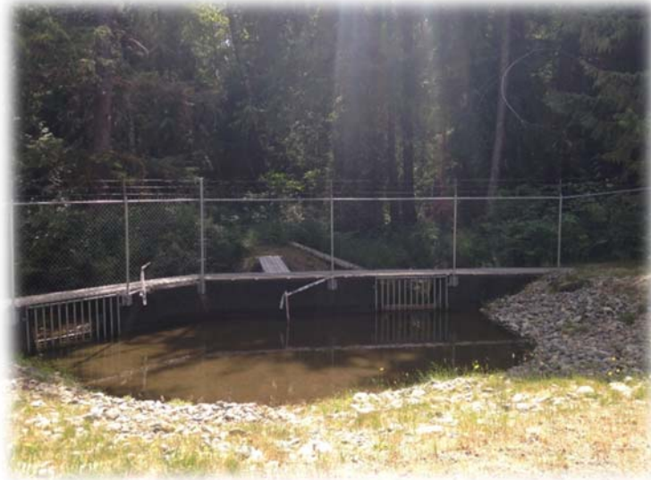
Infiltration Pond on Crocker Creek
