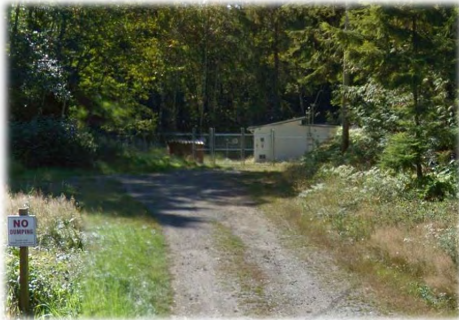
Water Intake Location and Pumphouse
