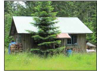
Vertical log cabin (caretaker's residence) in the northeastern corner of the park (RDN photo)
