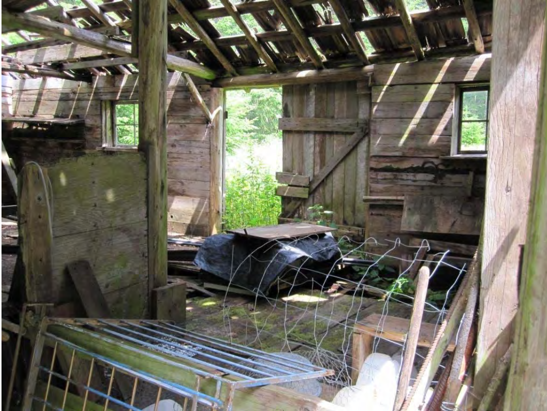
Interior view of Barn.
