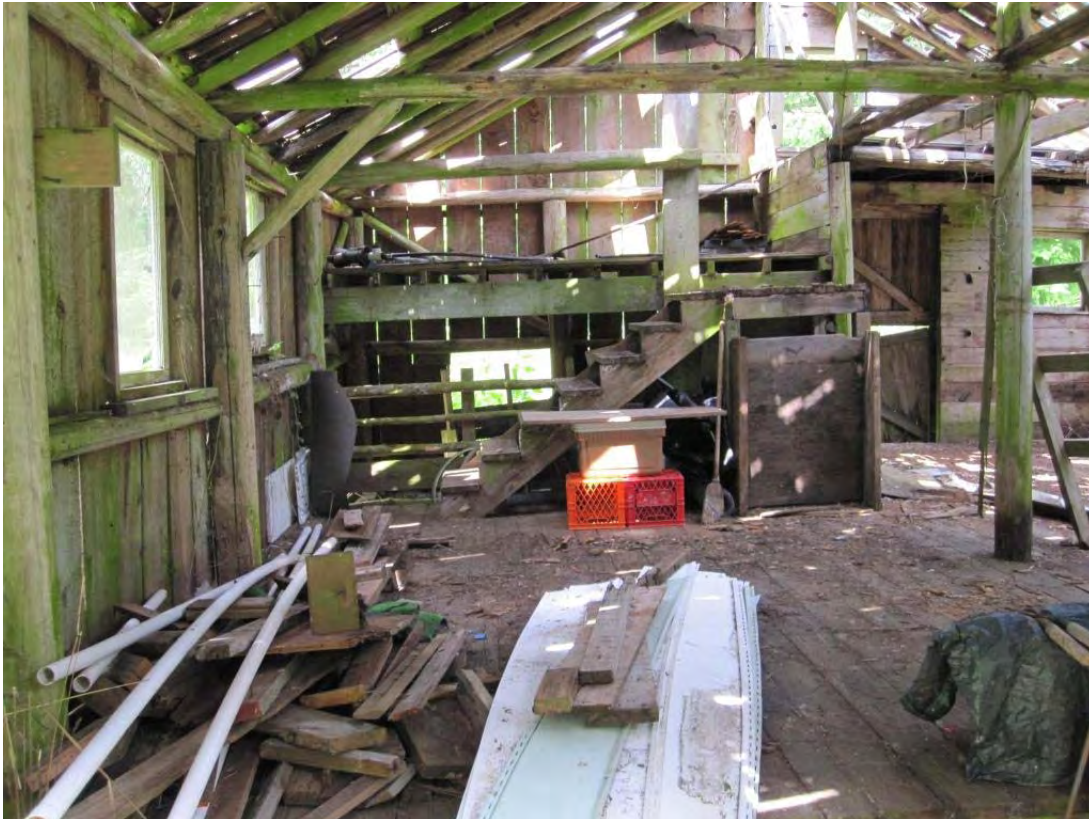
Interior view of barn.
