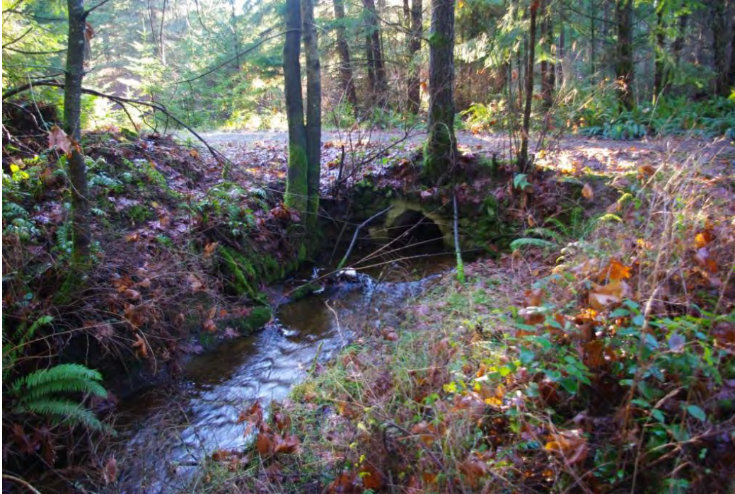
Photograph 13: Watercourse 3 where it flows under the park road in culvert.
