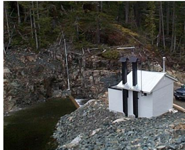
Arrowsmith Dam – Control Station
