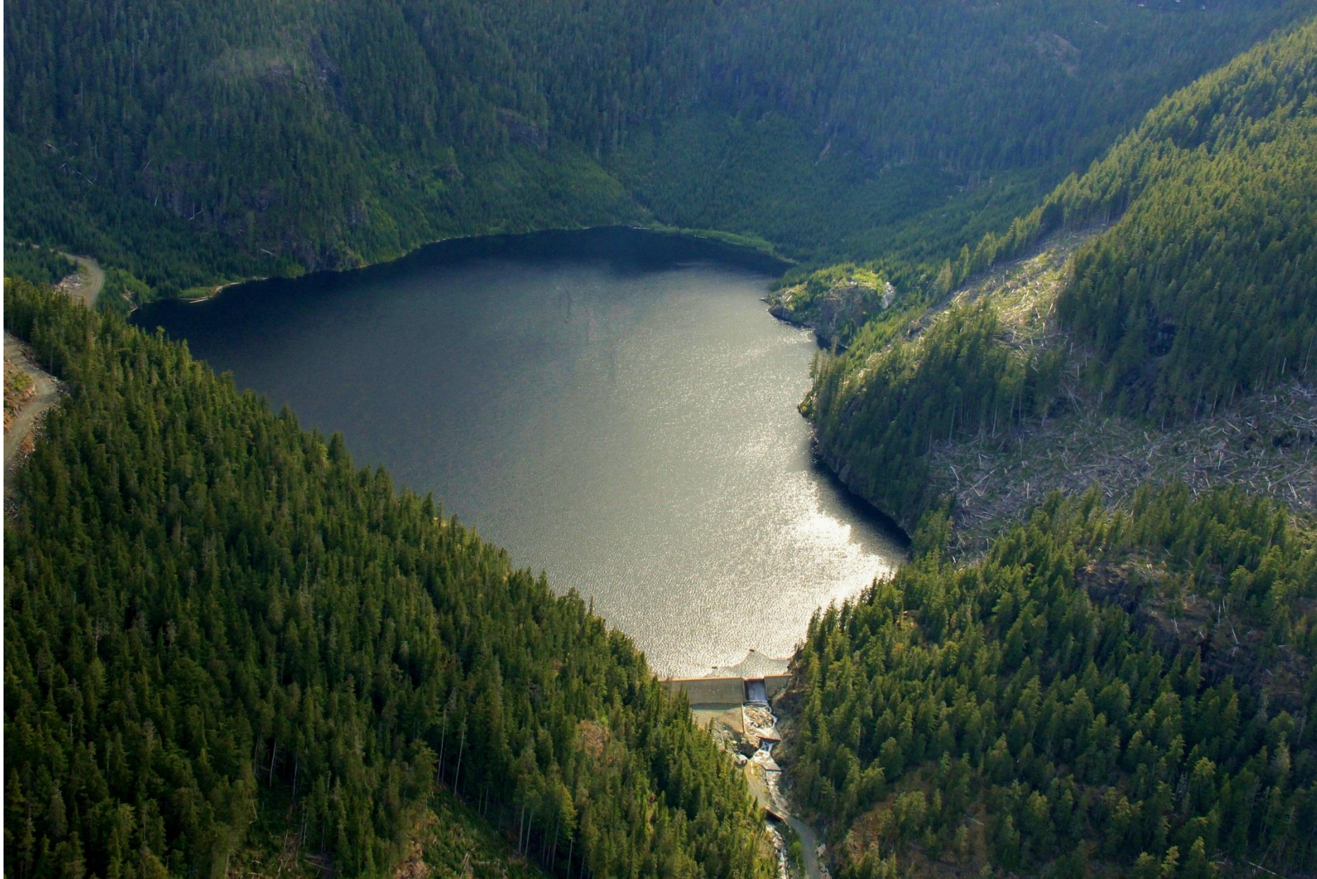
Arrowsmith Lake Reservoir (June 2013) - looking south
