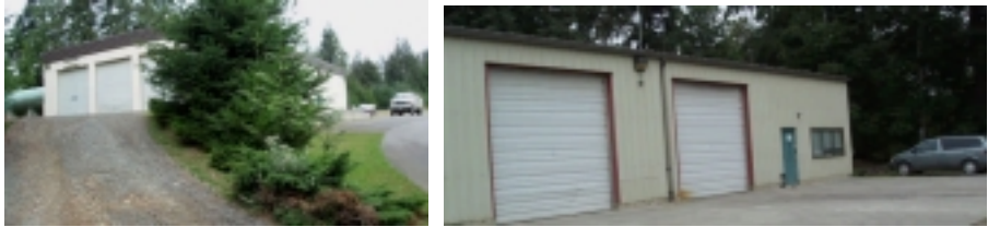
Photos. Gabriola Island’s two fire halls are equipped with generators.
