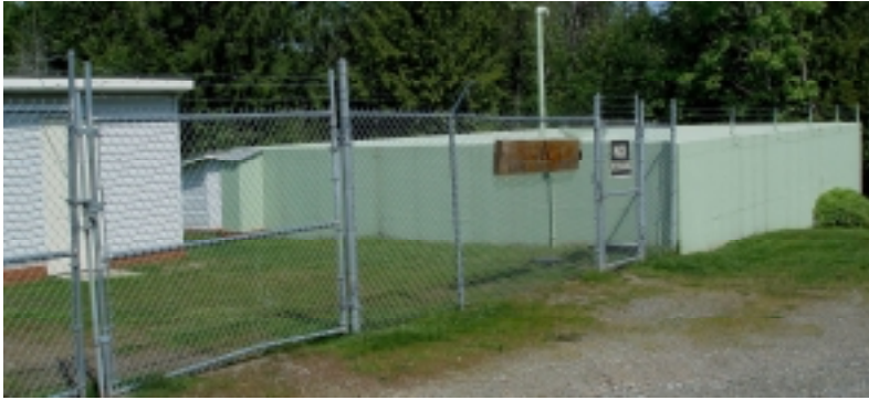
Photo 22. Qualicum Bay-Horne Lake Waterworks.
