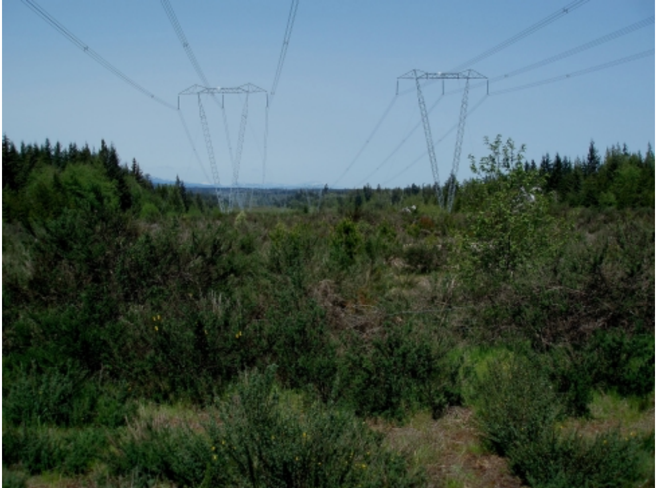
Photo 20. BC Hydro power line rights-of-way cut through Bow Horn Bay.
