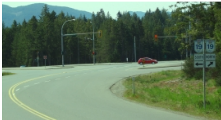
Photo 80. Inland Island Highway/Horne Lake Road intersection.
