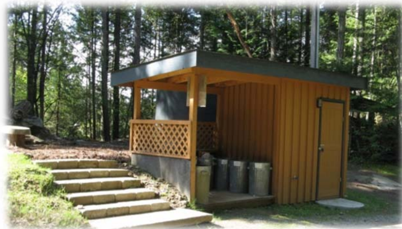
Descanso Bay Park Pumphouse (green cistern is located behind the pumphouse)
