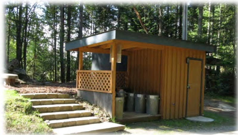
Descanso Bay Regional Park Pumphouse (cistern is located behind the pumphouse)
