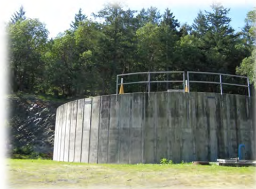
Photo of Fairwinds Reservoir No. 1
