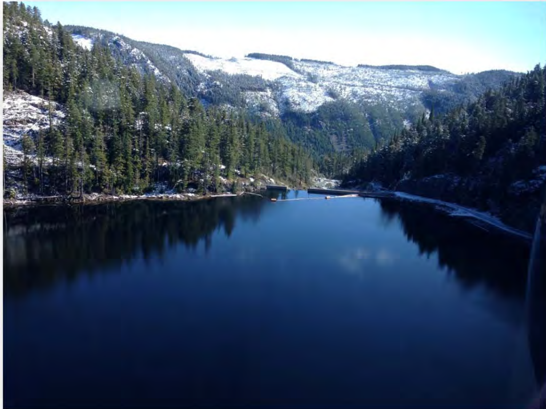
Arrowsmith Dam April 2014
