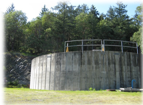
Photo of Fairwinds Reservoir No. 1
