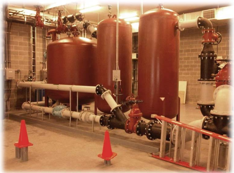
Completed Water Filtration Plant Filtration chambers shown
